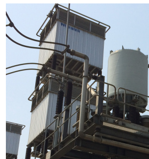
Figure 6 Spark Gap
